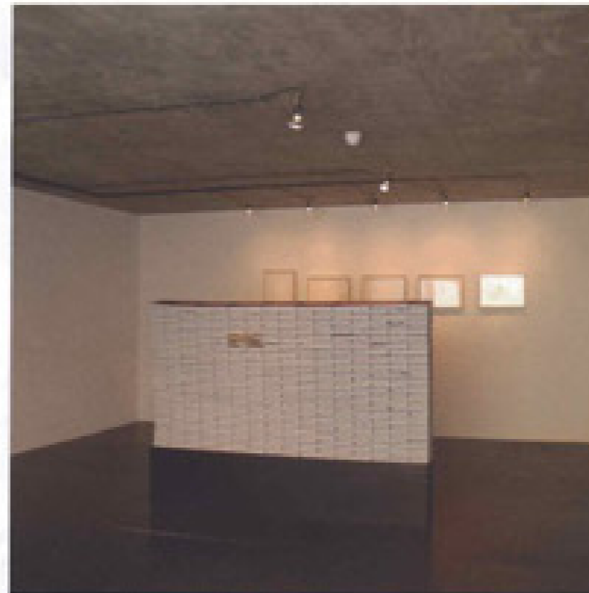
Hang 'em high The low ceiling height of the ground floor gallery space meant the lampholders could be suspended on short aluminium rods, in the downstairs gallery, however, they hang about 200mm from the ceiling
